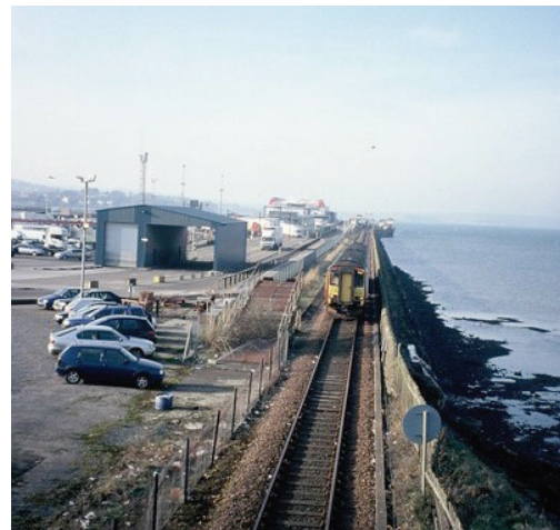
Stranraer: Public Transport Interchange site
